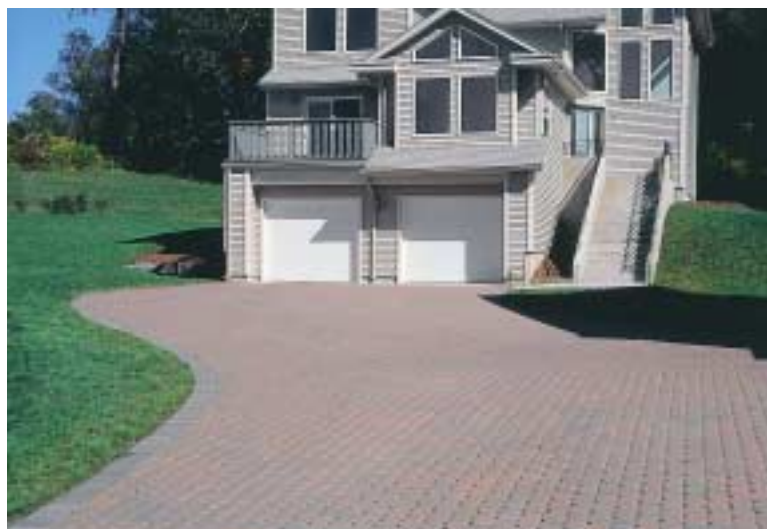
Glen Brook Green features shared Eco-Stone® permeable pavement driveways
