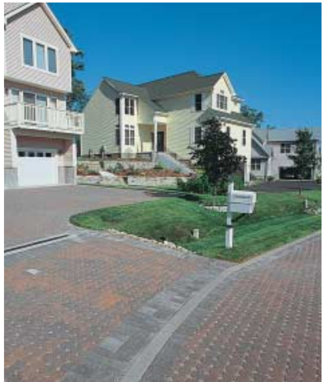
Grass swales provide additional runoff control, help filter sediment, and offer pollutant reduction capabilities
