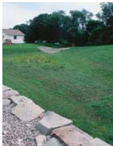
One of Glen Brook Green's vegetated bio-retention areas
