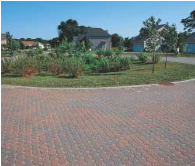
A "rain garden" is incorporated into the Eco-Stone® cul-de-sac
