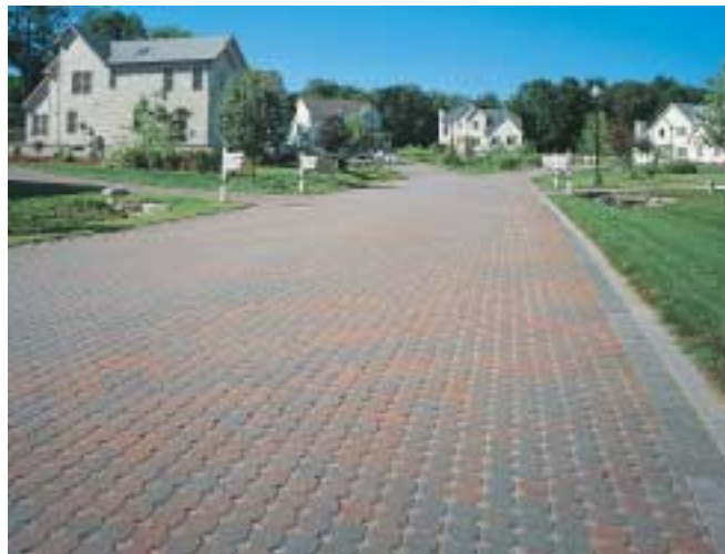
The Eco-Stone® permeable pavement streets and driveways remain in excellent condition after several winters
